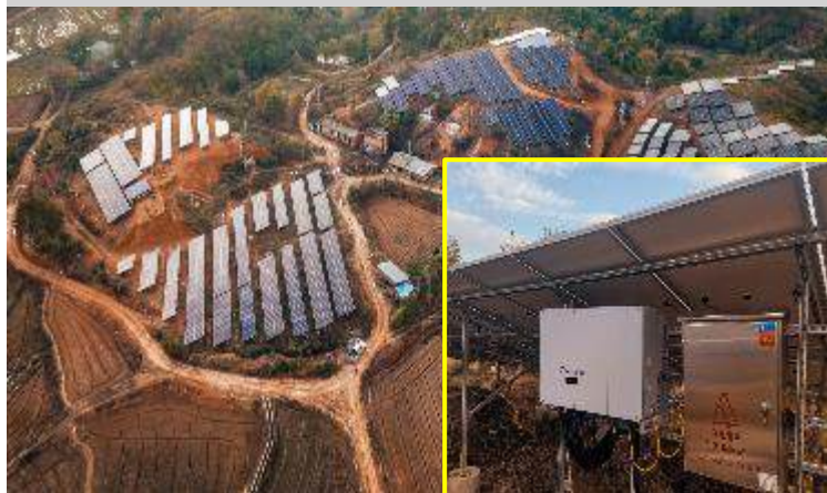
Ground Mounted 8 MW, 80/100/110/120kW inverters Suichuan, Jian, Jiangxi, China
